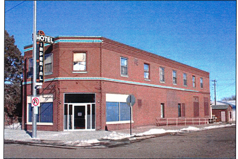
Photo 6: While sidewalks have been improved, some sections of curb and gutter, as well as street surfaces, need improvement, Site 3
