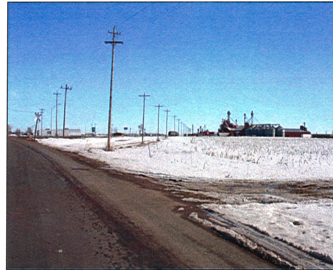
Photo 3: Inadequate pedestrian lighting combined with poor pedestrian infrastructure pose a danger to local citizens, as does the possibility of standing water, Site 2.
