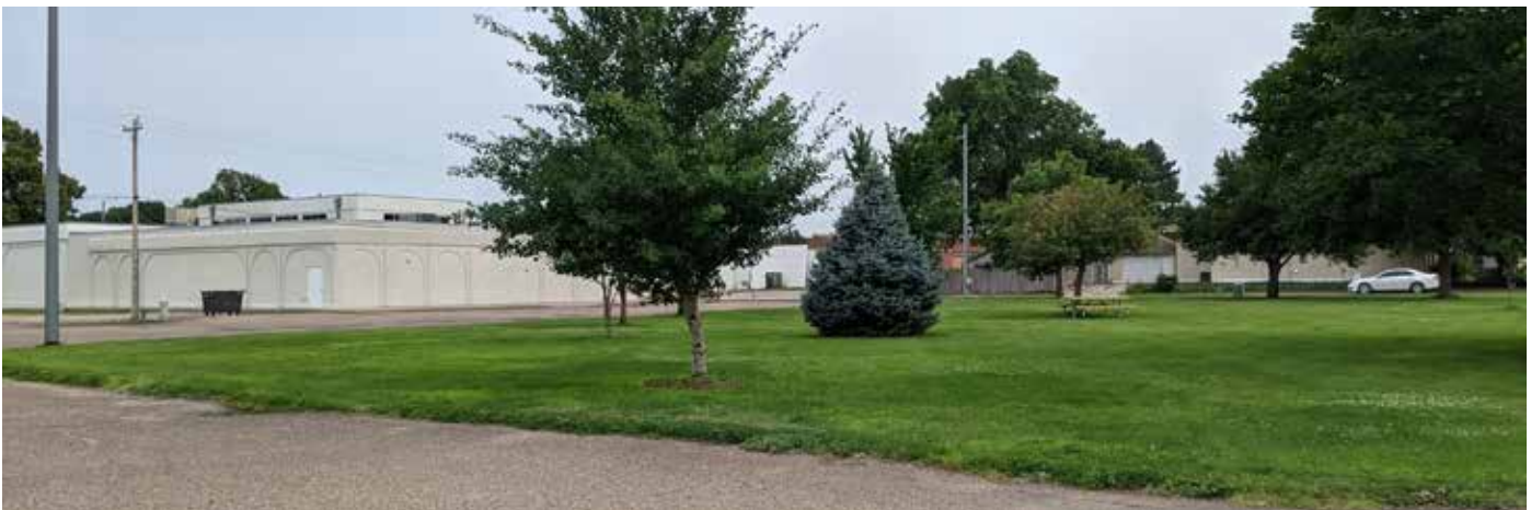
Existing condition from west parking lot entry, looking southeast toward Lied Imperial Public Library.
