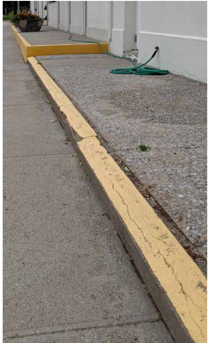
Elevation changes and lack of railings outside of both buildings on the site present accessibility concerns.
