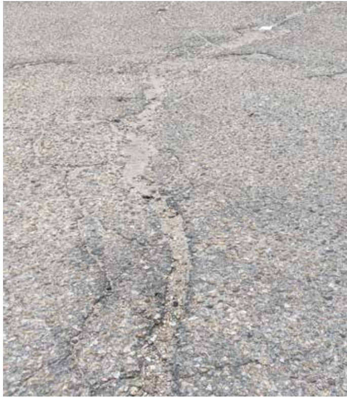
Large cracks exist in the existing parking lot.
