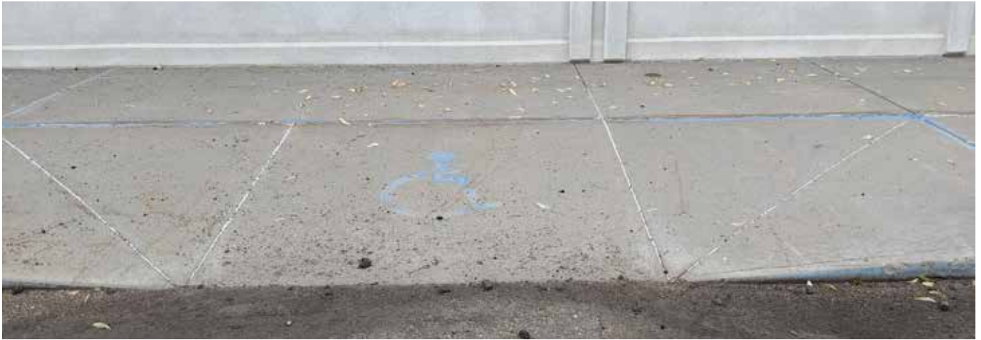
Sidewalk ramp located on west side of Lied Imperial Public Library
