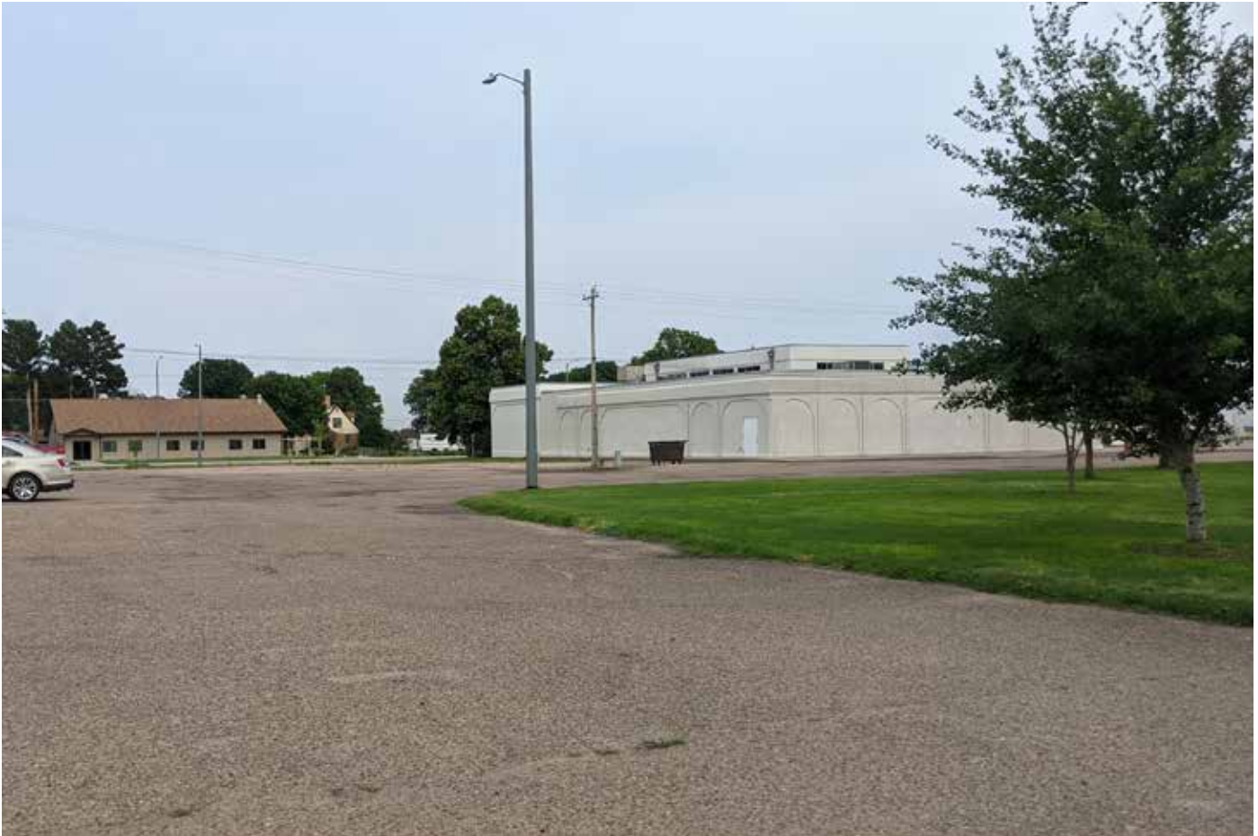
Existing condition looking southeast, toward Lied Imperial Public Library, from the west parking lot entry.
