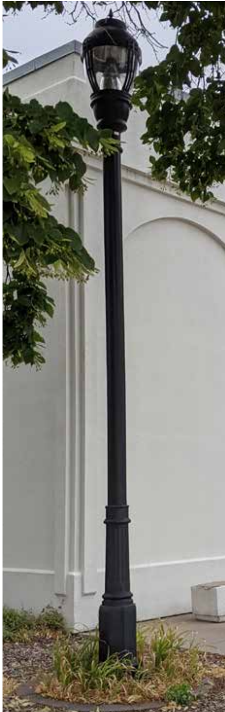
Existing pedestrian light post in front of Lied Imperial Public Library.
