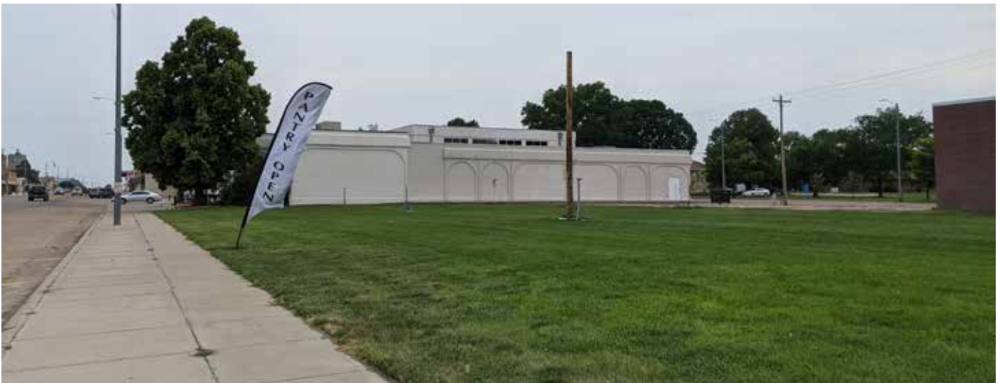
Existing condition looking south-southwest, toward Lied Imperial Public Library, from northeast corner of the site.
