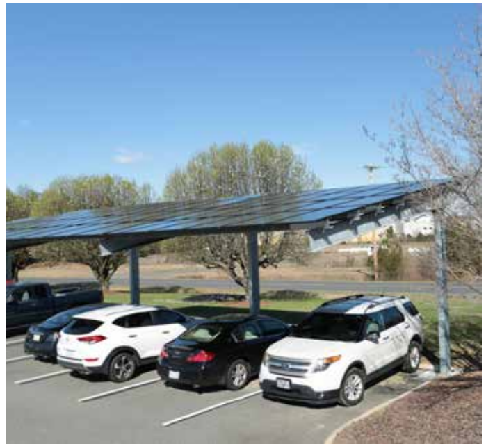
Example of car canopy with solar panels. (Image from https://preformed.com )
