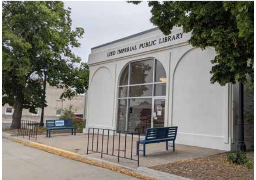
Front entry to Lied Imperial Public Library on east side of building.
