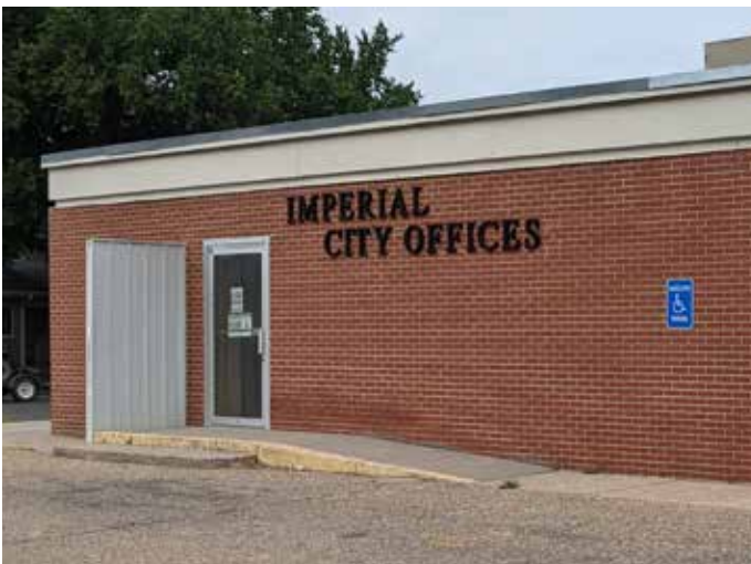
Elevation changes and lack of railings outside of both buildings on the site present accessibility concerns.
