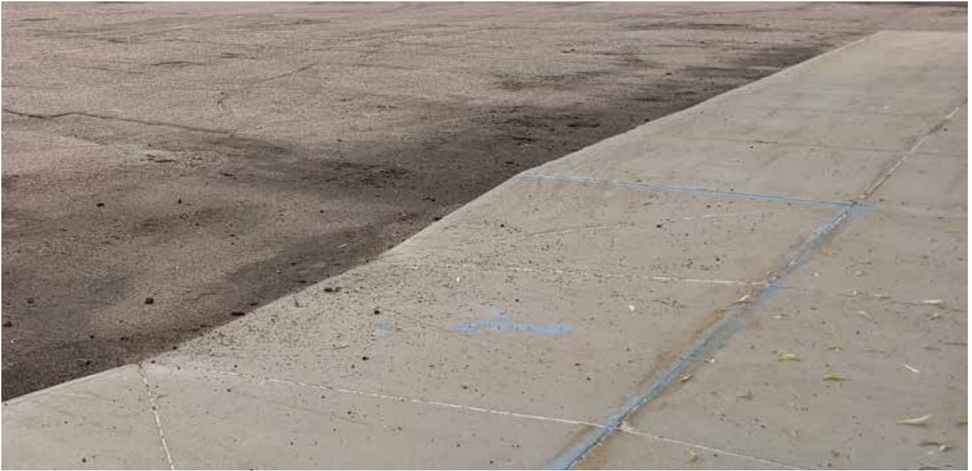
Existing ramp on west site of Lied Imperial Public Library.
